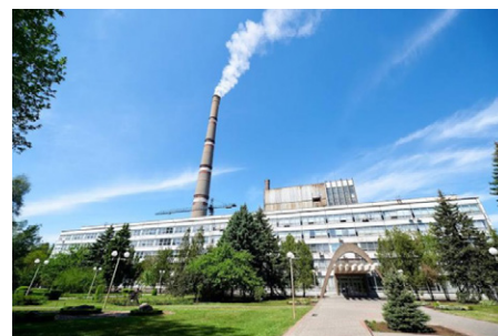
Figure 1: DTEK chose Honeywell to deploy BESS technology at its Zaporizhzhya power plant.
